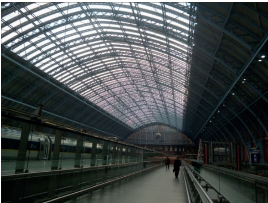
Figure 3: The roof of St Pancras station in London, reportedly constructed using self-cleaning glass
