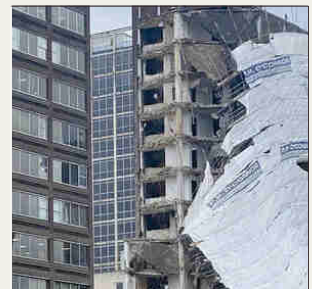
Scaffolding back in the news
